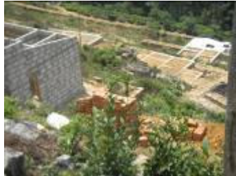
Foundations for new houses at Idulgashinna
